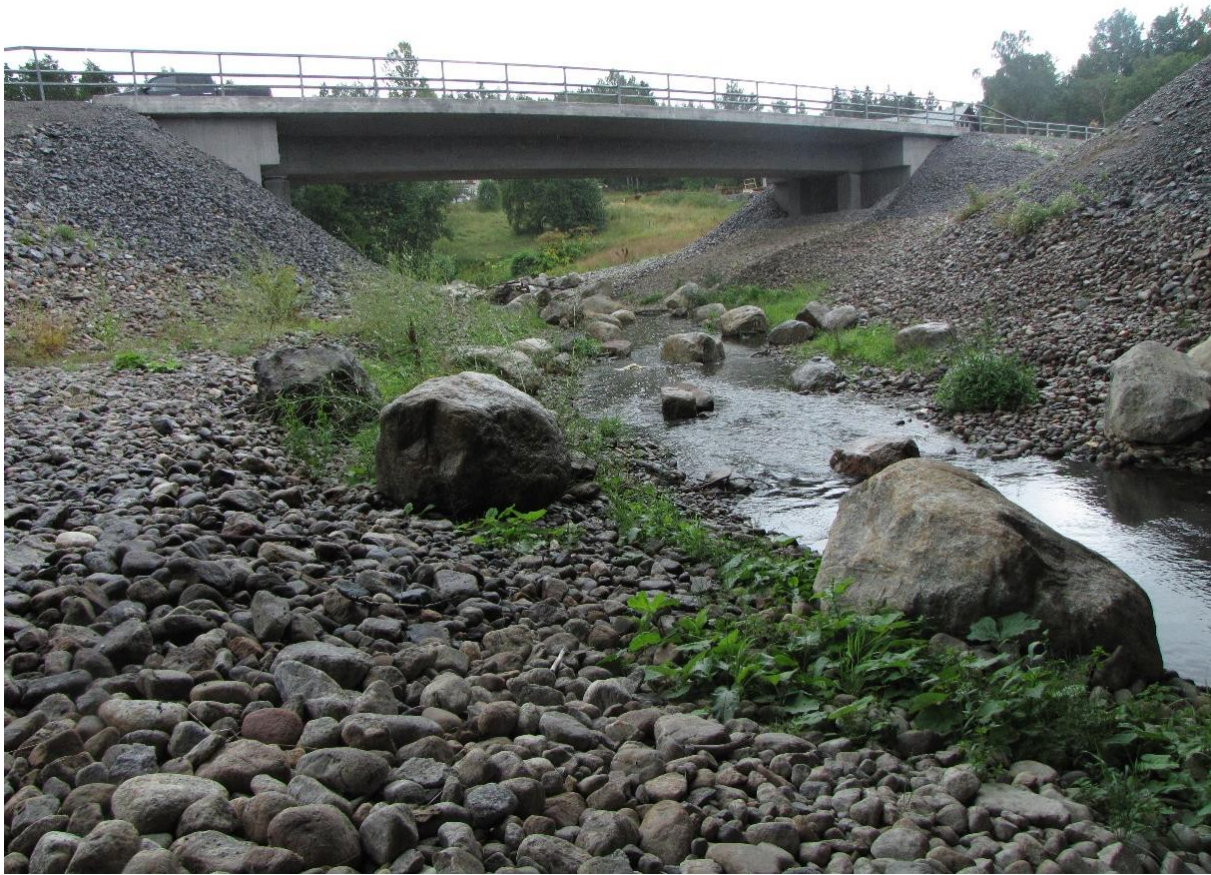
Figure 7.2: A creek restored in connection with a new road in order to create aquatic habitats, e.g. for spawning trout. Överfors, Province of Södermanland, Sweden, 2011.
