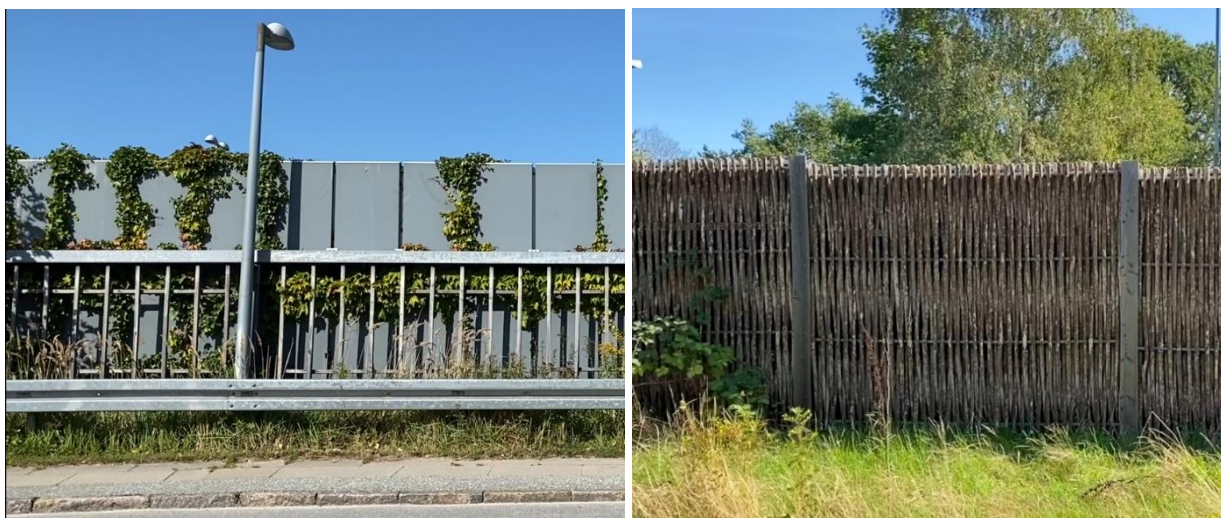
Figure 1: Examples of barrier design and surroundings affecting the perception of traffic noise annoyance.
