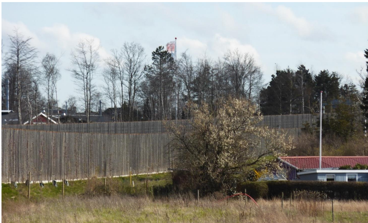
Figure 14: Wooden noise barrier adapting to the surroundings. It is designed in a way that is similar to the design and materials used in the local community.
