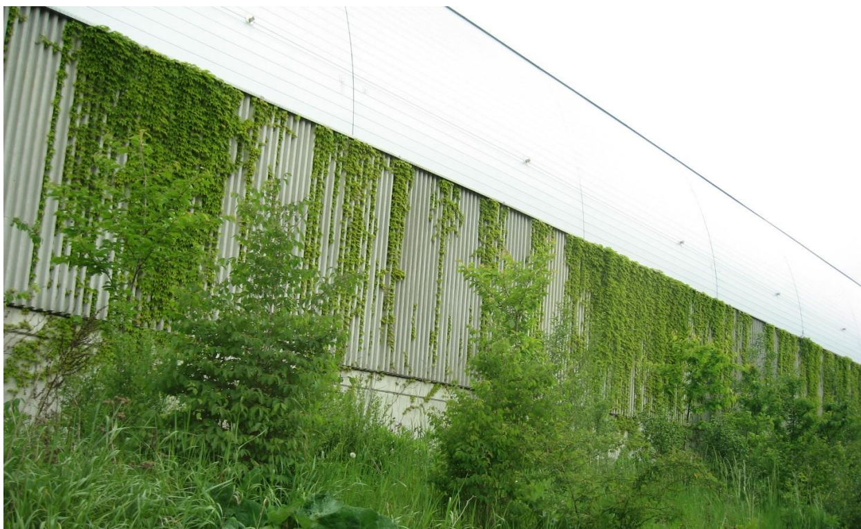
Figure 15: Greenery covering the lower part of a high noise barrier.
