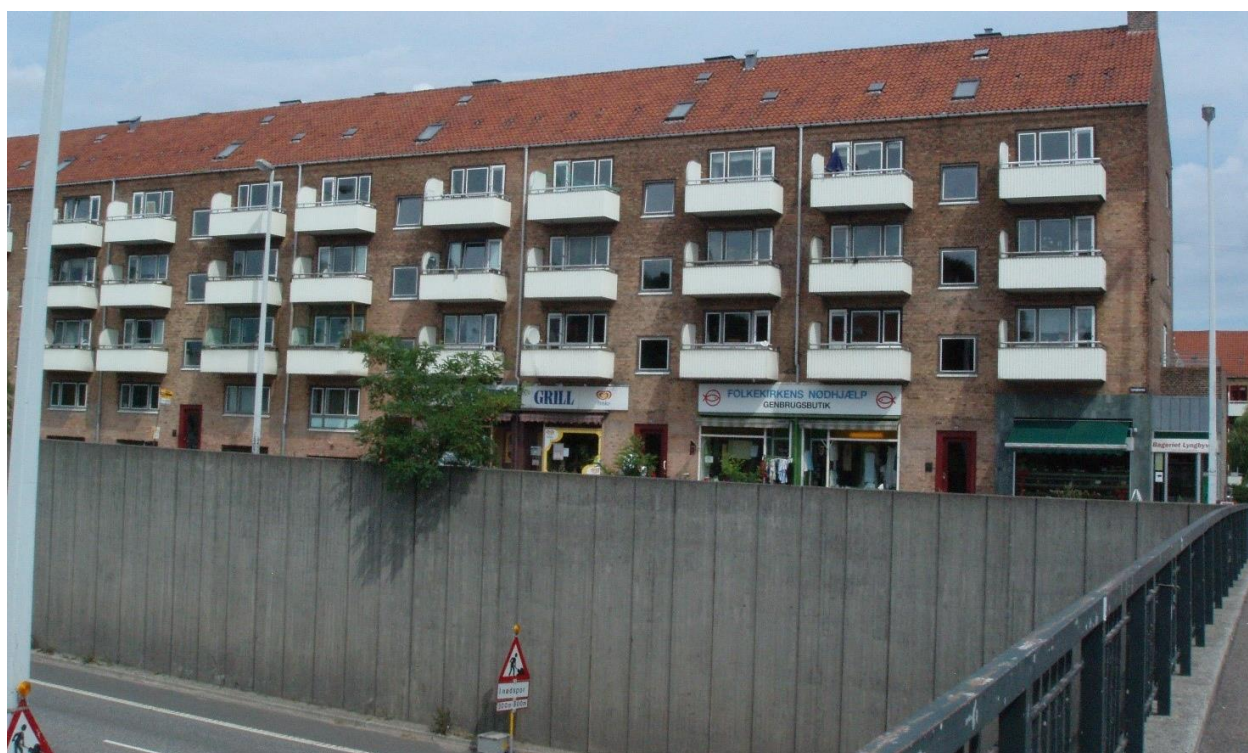
Figure 18: One facade facing the noise from the 6-lane motorway in the front, with chance to a quiet side on the far side. Typical two-room apartments, balconies suggesting living rooms on the loud side, giving a silent side for bedrooms.
