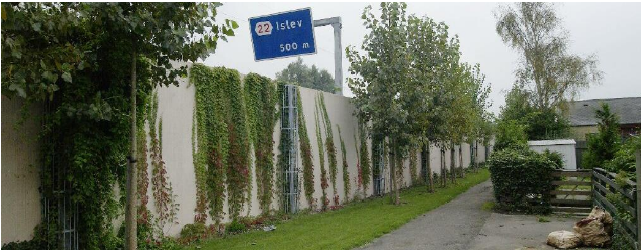
Figure 12: Noise barrier with greenery, reducing the visual impact. Possible negative influence on noise propagation!
