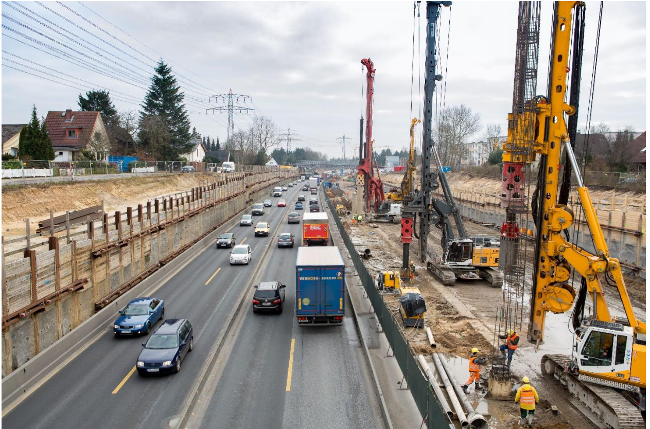
Figure 24: Construction site noise at a major motorway enlargement.
