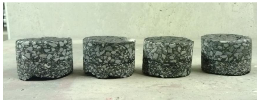
Figure 4. Asphalt cores collected from site trials
