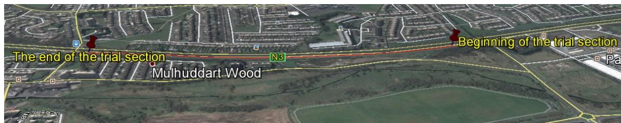
Figure 3-2: Satellite image of the trial road section
