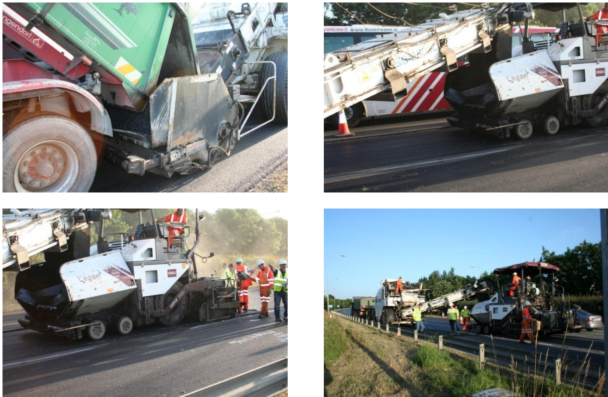
Figure 3-4: Paving process of the trial section
